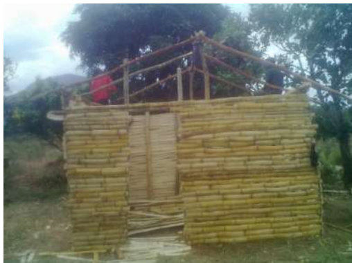
Fig 1: Mushroom house construction
