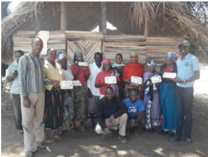
Three Mushroom houses constructed
